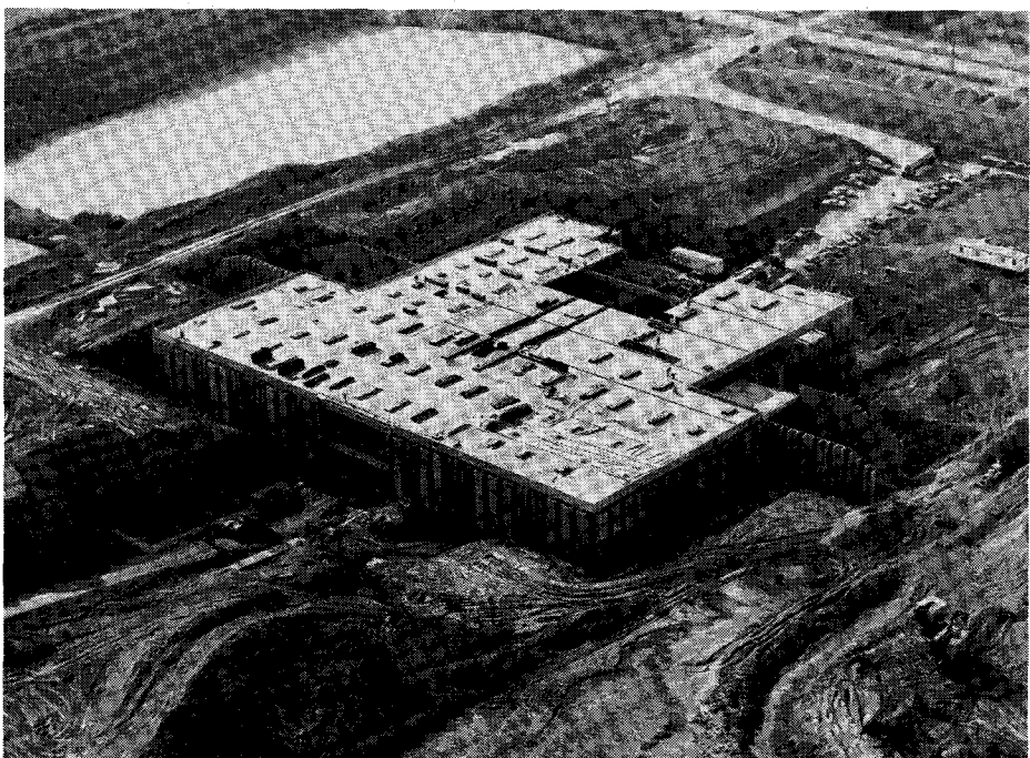
Fig. 3. Aerial view (looking from the north) of partially completed structure showing excavation (backfill) amidst mined terrain.
