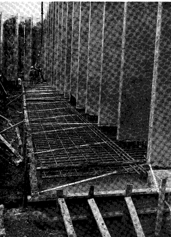
Fig. 8. Precast concrete retaining wall base connection. Note that heel portion of footing was cast in place (see Fig. 7).
